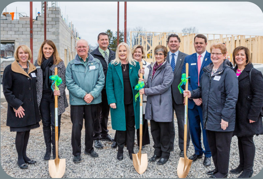
Members of Ability Partners, Inc., Ability Partners Foundation, Golisano Foundation, AutismUp, Wegmans, and Al Sigl Community of Agencies prepare for breaking down barriers with their ceremonial groundbreaking (above).
